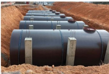
· Product: Double wall tank 50,000L - 6 units / Installation site: Storage site in Bitgaram-dong, Naju-si, Jeollanam-do
