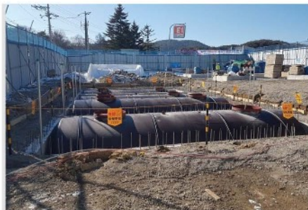
· Product: Double wall tank 50,000L - 4 units / Installation site: Anheung-myeon, Hoengseong-gun, Gangwon-do <Hoengseong service area - Chuncheon direction>
