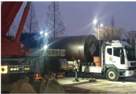
· Product : Double wall tank 40,000L - 4 units / Installation site : Daejeo-dong, Gangseo-gu, Busan <Eunma Petroleum>
