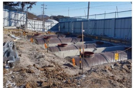
· Product: Double wall tank 50,000L - 4 units / Installation site: Anheung-myeon, Hoengseong-gun, Gangwon-do <Hoengseong service area - Chuncheon direction>
