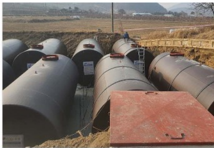
· Product: Double wall tank 50,000L - 14 units / Installation site: Gamgok-myeon, Eumseong-gun, Chungcheongbuk-do <Sangpyeong gas station>
