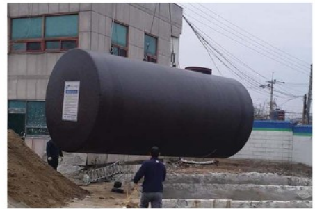
· Product : Double wall tank 40,000L - 4 units / Installation site : Daejeo-dong, Gangseo-gu, Busan <Eunma Petroleum>
