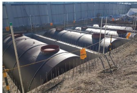
· Product: Double wall tank 50,000L - 4 units / Installation site: Anheung-myeon, Hoengseong-gun, Gangwon-do <Hoengseong service area - Chuncheon direction>
