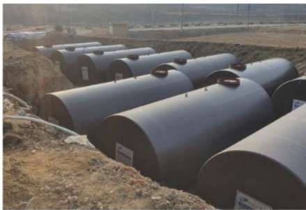
· Product: Double wall tank 50,000L - 14 units / Installation site: Gamgok-myeon, Eumseong-gun, Chungcheongbuk-do <Sangpyeong gas station>
